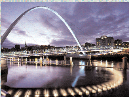
Gateshead Millennium Bridge. Photograph courtesy of Gateshead Council. Image by i2i Photography.
