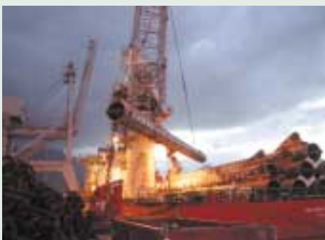
Loading 2m x 30m mooring piles weighing 100 tonnes
