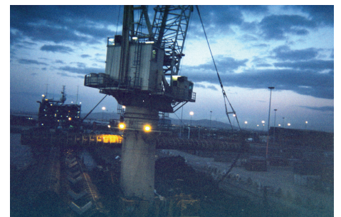
Crane on diverless construction vessel, Cape Town
