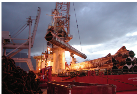
Loading 2m x 30m mooring piles weighing 100t
